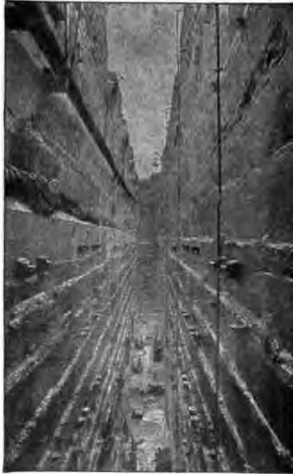
Fig. 125. Channeled Walls of Wheel Pit.
